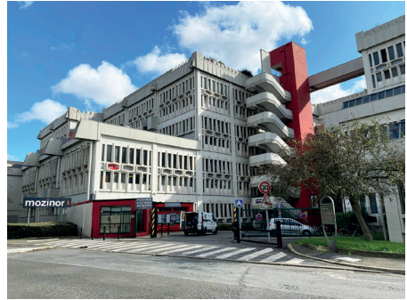
© figure 4, Usine Mozinor, Montreuil
